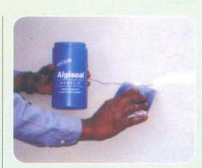
takes up to one day) apply the sealant once again. (For roof cracks try to maintain convex surface at the top) Applying the sealant twice is recommended for waterproofing repairs. Wait till the second coat dries for subsequent waterproofing repairs. For internal wall cracks, Algiseal Acrylic needs to be applied 3 times and allowed to dry for uniform appearance on the walls.
