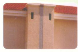
depth of the sealant should be equal to half width but subjected to minimum of 6 mm and maximum of 12 mm.
